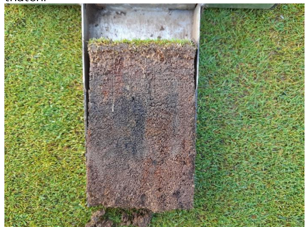
Photo 6: The newer USGA greens were thatchy and had black layer in the profile. These types of green are notorious for building thatch and are also very susceptible to black layer.
